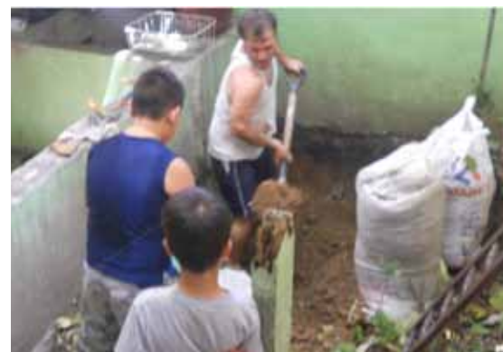
Digging the hole for a water retaining tank.
